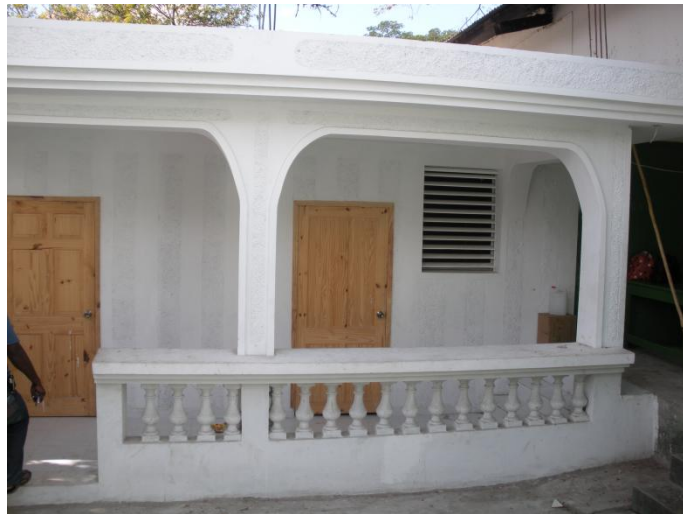
The outside view of new isolation rooms in Hinche
