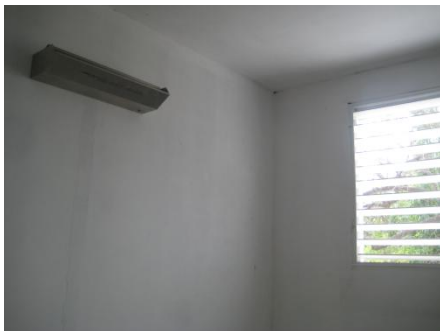
A recently installed UV Light and improved ventilation inside an isolation room
